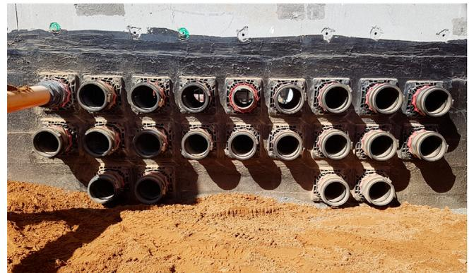
KME trialled three to begin with, the builder then approved the system and completed another layer of the membrane. New core-holes were drilled then another twenty two HSI 150-DFK and system covers were installed after early success and ease of installation.
