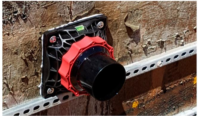
HSI system cover is then simply attached via the bayonet system to the DFK and tightened by the red clamping nut.
