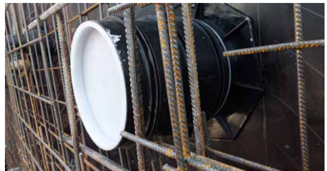
UFR in formwork
