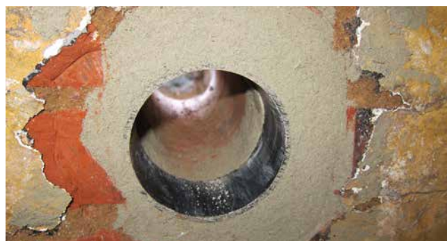
SFR subsequently incorporated into the masonry
