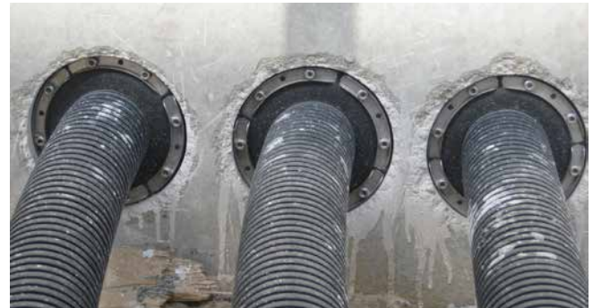
Detailed view: Clip ring/seal
