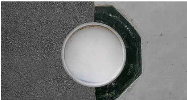
concreted UFR with PMBC
