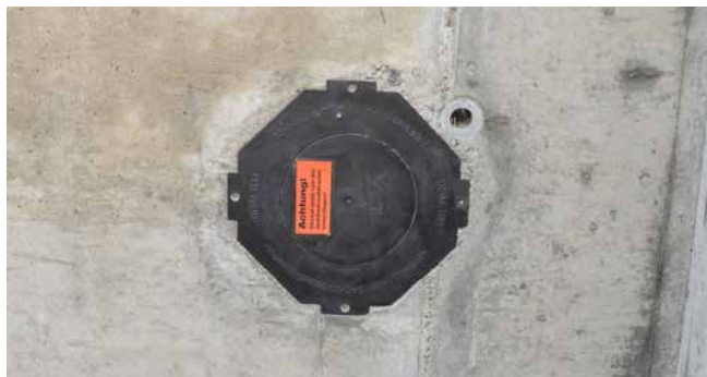
Practical picture of UDM/UDME in concreted wall
