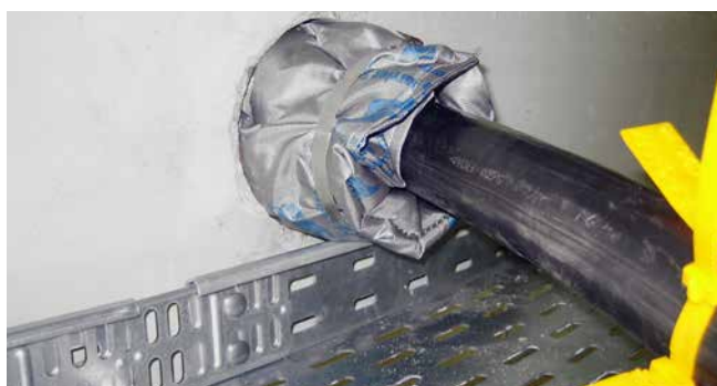
HSS - installation in core drill hole with HRD press seals
