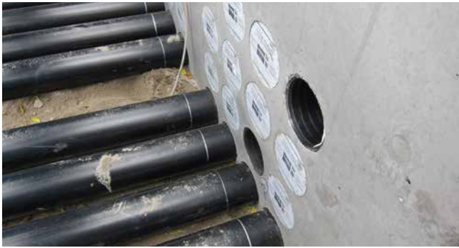
HSI150 GSM Varia applied as a block
