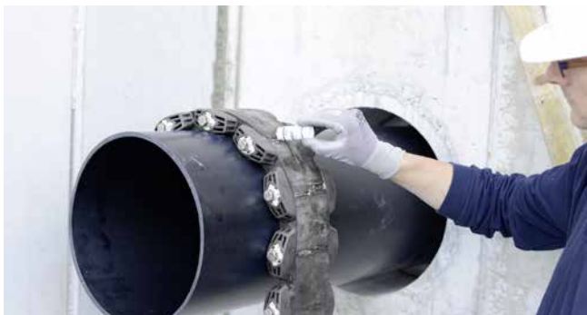
GKD400 - installation preparation with lubricant GM
