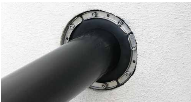
HSD200 1x159 b20 A2/EPDM55 "shaft seal"
