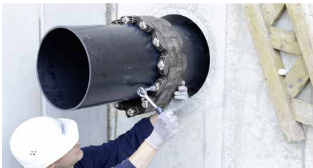
GKD400 - tightening of segments
