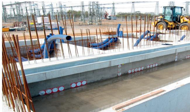
Flexible cable duct systems KES-M 150 using Hateflex 14150 and KES-M 90 using Hateflex 14090 are being laid.
