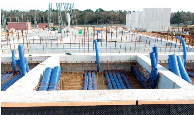
Cable ducts are being laid and connected to the wall inserts using sleeve method.
