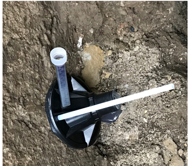
A white filling hose inserted in the building entry allows any air to escape, while butyl tape ensures a tight connection between the wall surface/building seal and the flange.
