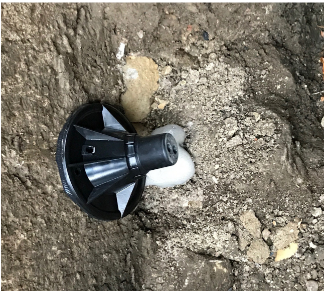
The expanded two-component resin compensates any irregularities in the wall, creating a seal that is both gastight and watertight.
