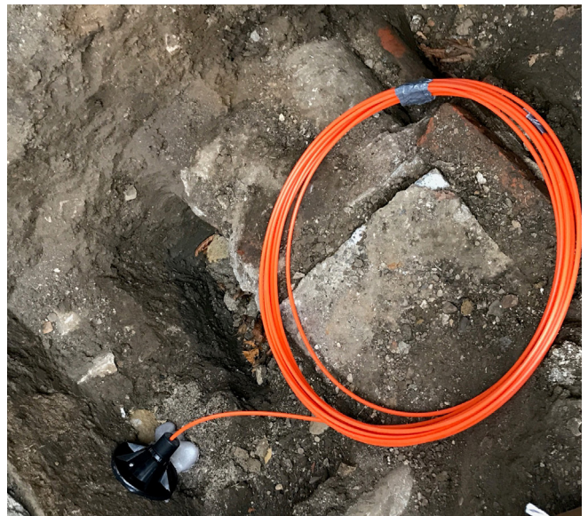
The speedpipe with a diameter of 7-10 mm can then be inserted properly into the GFH 30.
